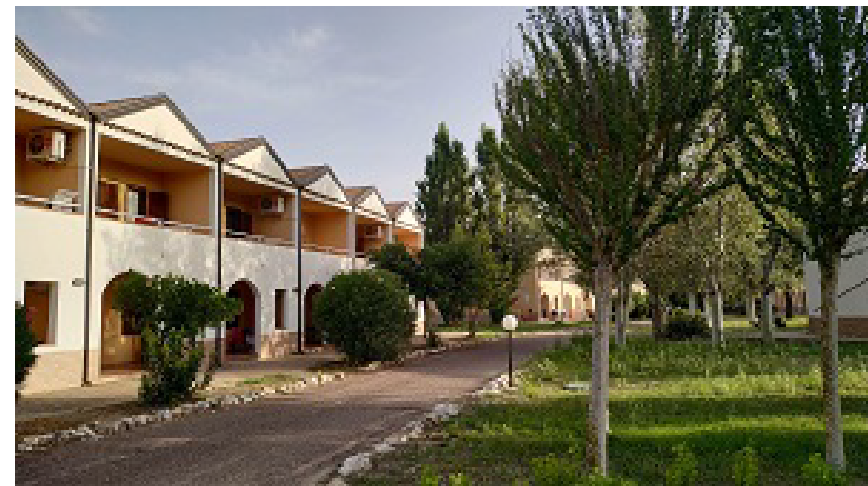
EXTERNAL STRUCTURE OF THE ACCOMMODATION COMPLEX
